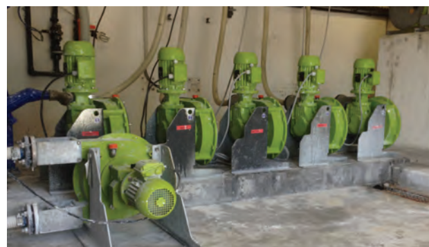
ALHX40 for lime milk in wastewater treatment
