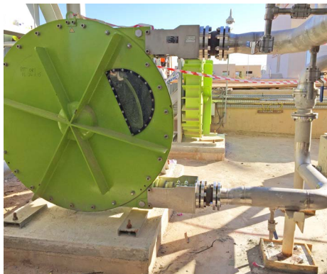
ALH125 pumping concrete
