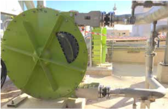
ALH125 泵送混凝土
